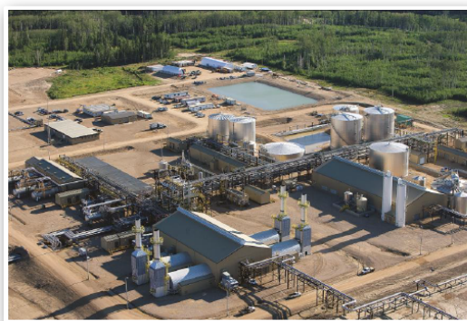
Surmont 1 Central Processing Facility
