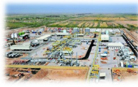
First Phase Installations of Halfaya Oilfield Centralization Treatment Station
